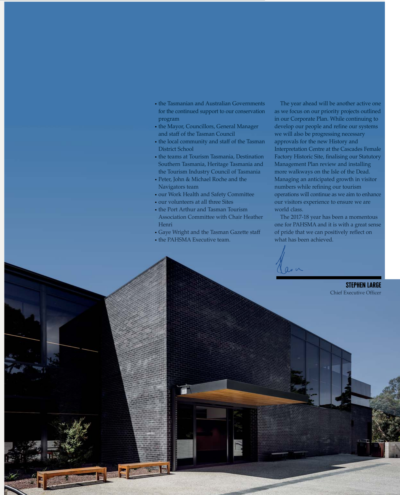
New Visitor Centre at Port Arthur Historic Site Image: Adam Gibson courtesy JAWS Architects
